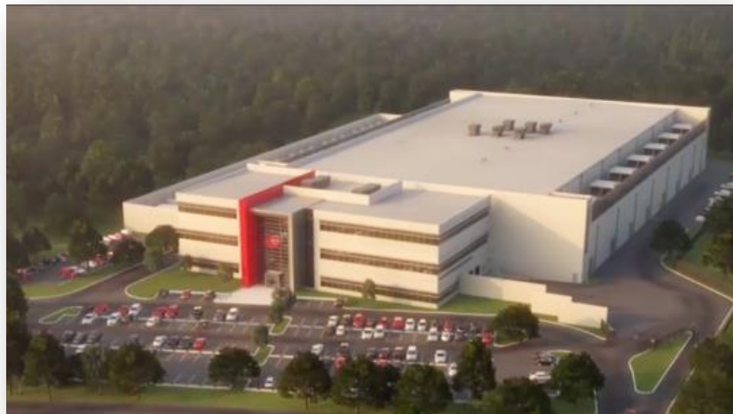
QTS Datacenter – Ashburn, VA
