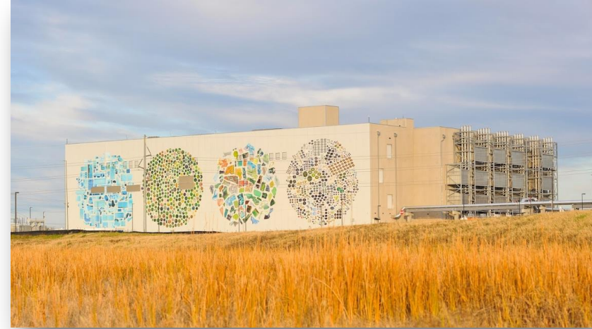
Google Datacenter – Mayes County, OK
