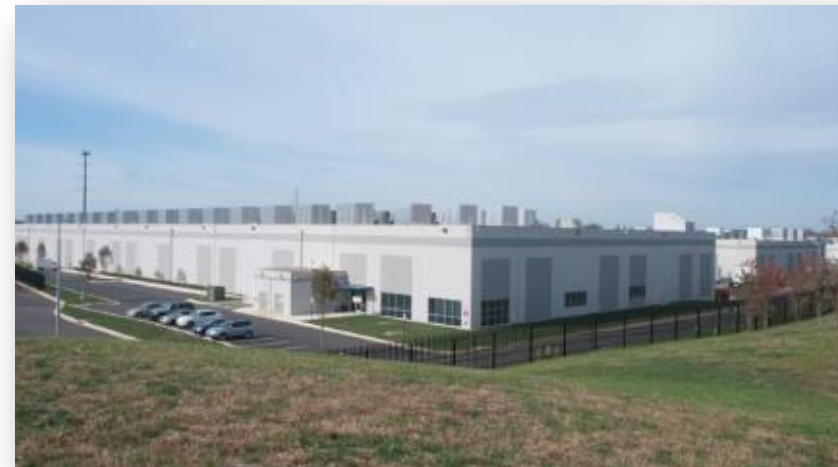
AWS Datacenter – New Albany, OH
